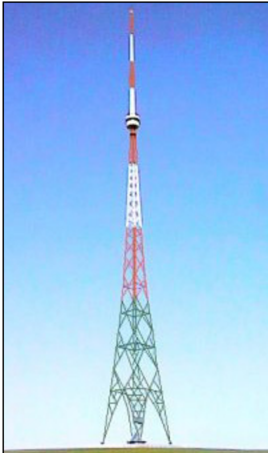
Figure 1: Switzerland's National AM Radio Station Beromünster Constructed in 1931 as an independent voice against the Nazi propaganda of Germany to the displeasure of Adolf Hitler. The station broadcasted AM signals until 2008.
